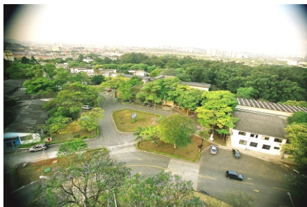
Figure 17. Aerial view of the Materials Science and Technology Center (CCTM-acronym in Portuguese)
